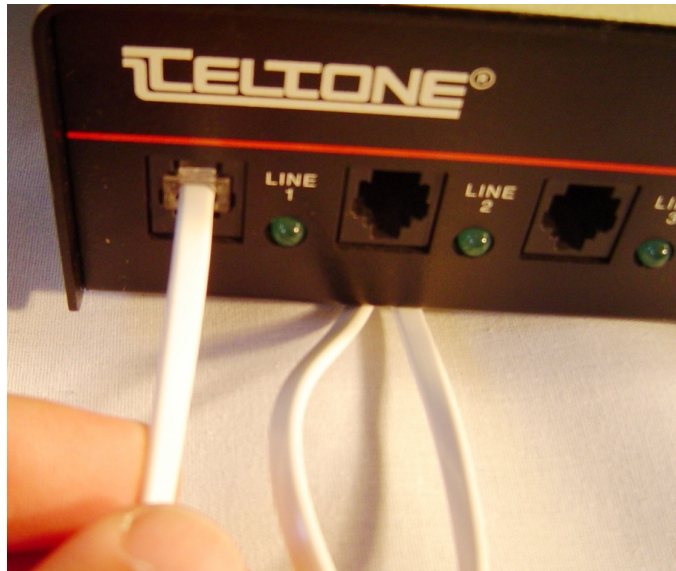
Figure 3 RJ-11 Connection to line simulator
